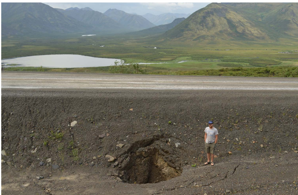
Fig. 3. A recurring sinkhole in the Dempster Highway embankment due to ground water flow at YT km 82 (2017).
