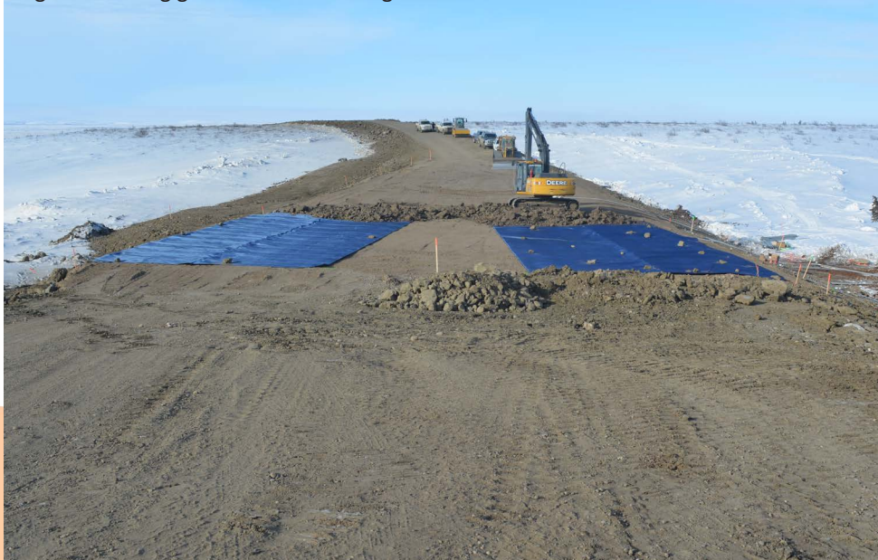
Fig. 19. Wicking geotextiles laid during construction of a reinforced section of the ITH.
