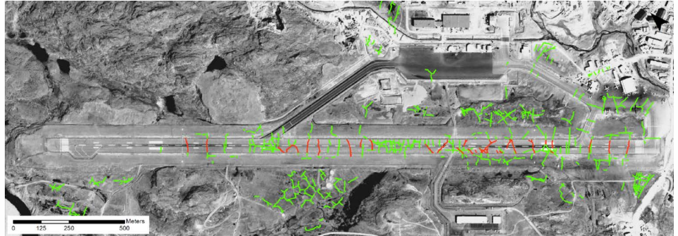
Fig. 24. Thermal contraction cracks mapped at Iqaluit Airport (green). Active cracks in the runway inherited from the original terrain conditions are shown in red (2010).
