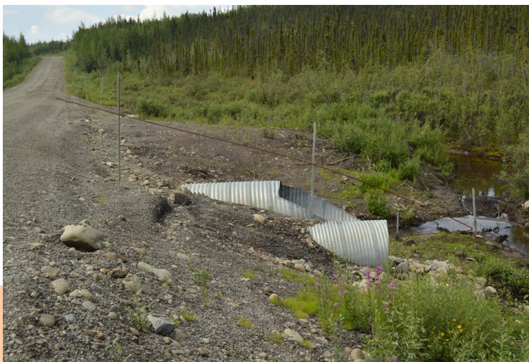
Fig. 2. Left: new culvert installed at YT km 32, Dempster Highway in the North Klondike River Valley after failure of the infrastructure due to ice blockage in 2014. Photo taken in 2017. Right: failure of the culvert due to icing development two years later (2019).
