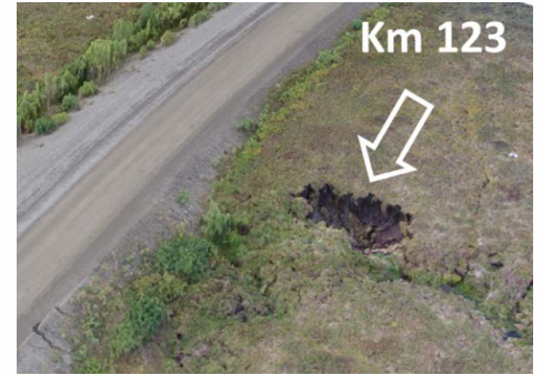
Fig. 26. Sinkhole forming due to thermal erosion at km 123, Dempster Highway.
