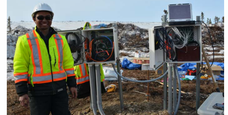
Installing sensors at the ITH test section, 2015.
